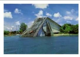
The foundation plinth with no shear reinforcement, 8.38 m deep, supporting a bridge pier, failed by shear because of one-sided riverbed scouring by flood. The size effect factor for shear was about 0.18.
