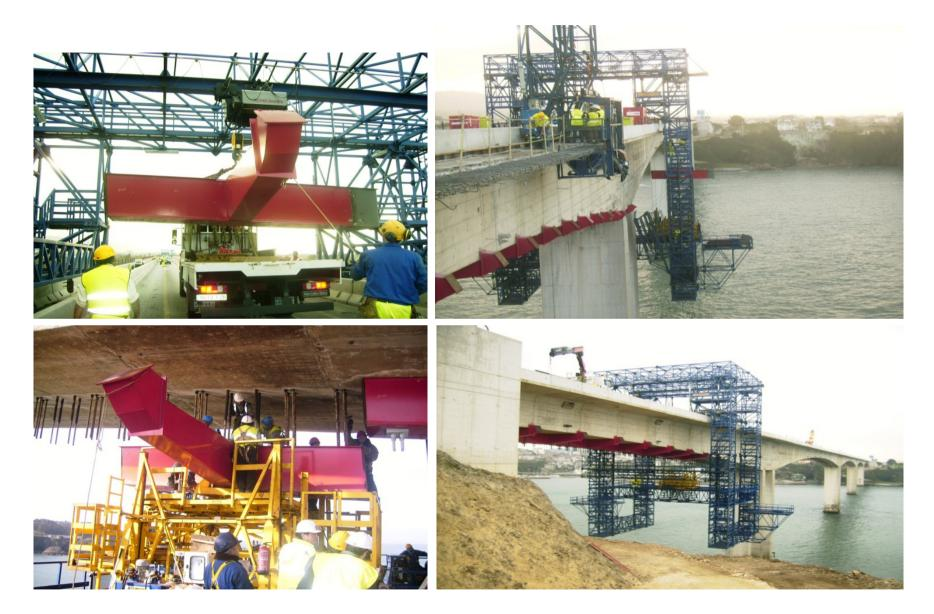
Execution of the steel structure under the existing superstructure
