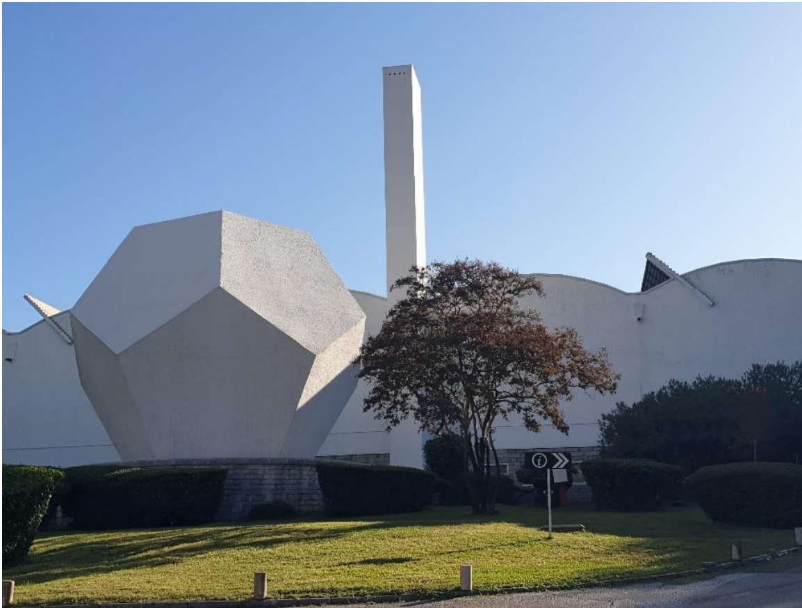
Torroja Institute, Madrid
