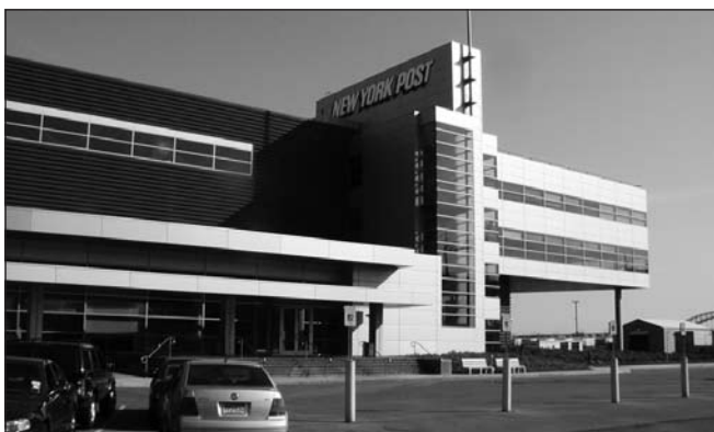
8. ábra: New York Post Printing Plant, NYC
