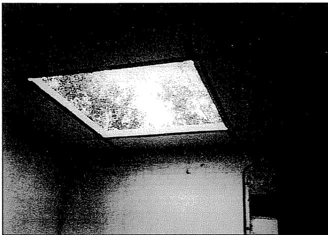
**Fig. 8** Strengthening around an opening in a reinforced concrete slab at ZOLTEK Rt. in Nyergesújfalú, Hungary. (Date: Aug. 1998. Strengthening strips: Sika CarboDur M1214-25 m. Designer: Dr. Rita Kiss and Akos Sapkás. Exec: Fischer-bau Ltd.)
