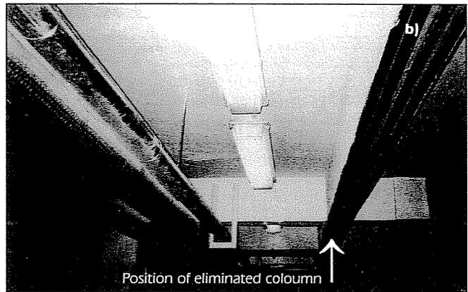
**Fig. 4** Strengthening of a reinforced concrete beam owing to the elimination of an intermediate column in the Stollwerck Chocolate Fabric in Budapest (Date: July 1996. Strengthening strips: Sika CarboDur S512-44 m. Designers: Dr. György L. Balázs, Dr. István Hamza, Dr. György Visnovitz, Exec: ISOPLAN Ltd. a) Elevation b) Photo after strengthening
