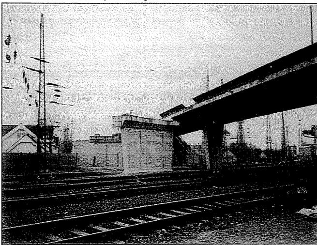
**Photo 3** New pier under construction next to the existing flyover
