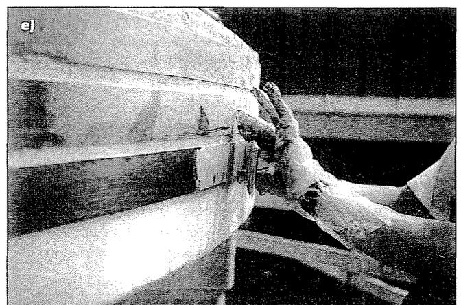
**Fig. 6** Strengthening of a grain silo in Berettyóújfalú, Hungary, owing to the corrosion of circular prestressing tendons (Date: June 1997. Strengthening strips: Sika CarboDur S612-152 m. Designer: Dr. György L. Balázs. Exec: Isobau Rt.)
