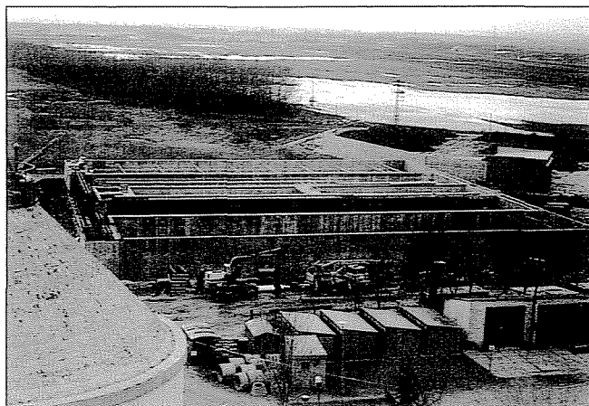
Fig. 7 Construction process of the block biological treatment structure before finishing
