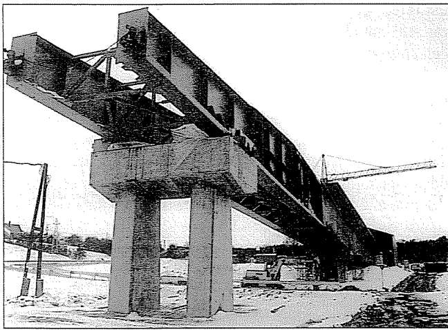
Fig. 4 Construction deck of Viaduct I
