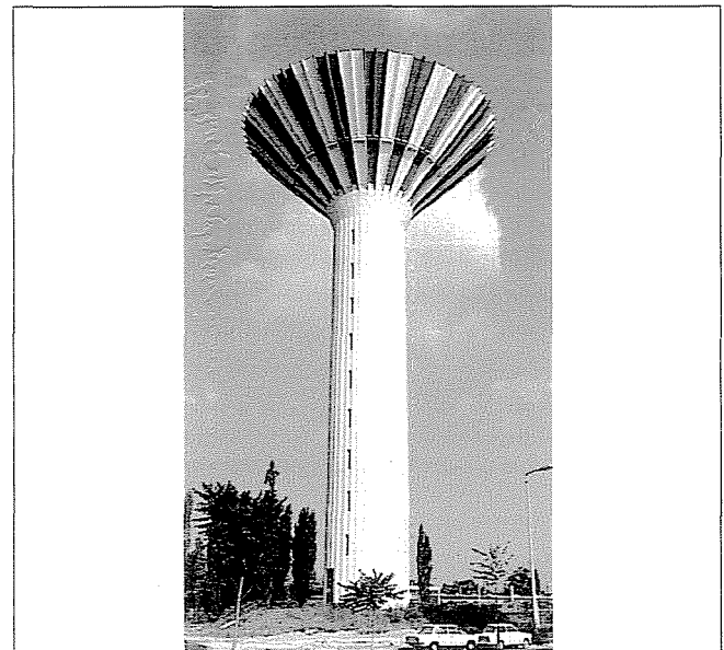
Fig. 9 Slip-formed stem and precast tank for water tower
