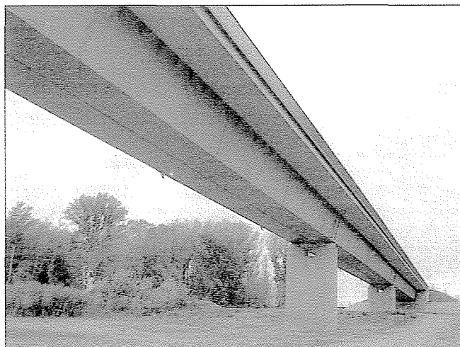
Fig. 3: Danube bridge at Szekszárd, view of flood bridge
