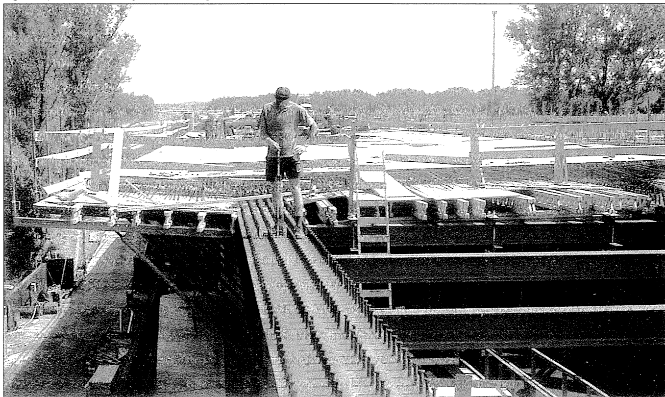
Fig. 9: Deck slab of Tisza Bridge at Oszlár during construction
