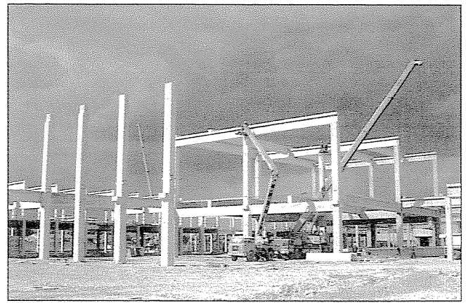
Fig. 6: IBIDEN 2 Construction of the hall framework with intermediate floor
