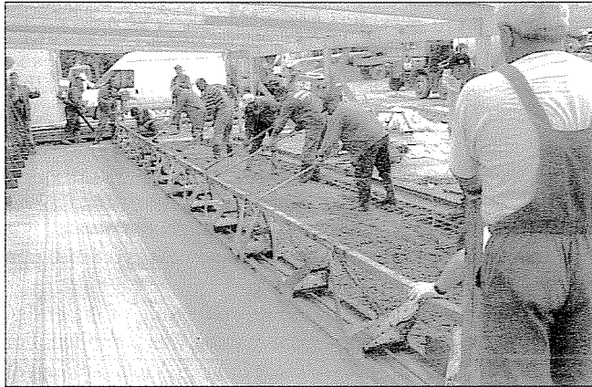
Fig. 10: Surface finishing with Tremix SVE beam screed
