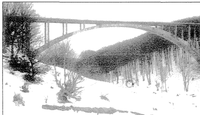
Fig.1: Viaduct at Mecseknádasd
