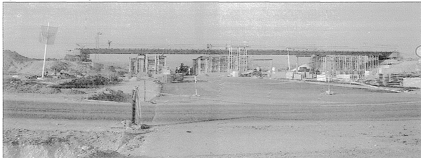
Fig. 8: General view of the bridge under construction
