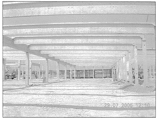
Fig. 2: IBIDEN 2 Hall framework exterior
