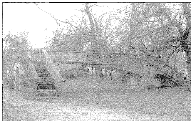
Fig. 2: The first concrete bridge (designed by Robert Wünsch)
