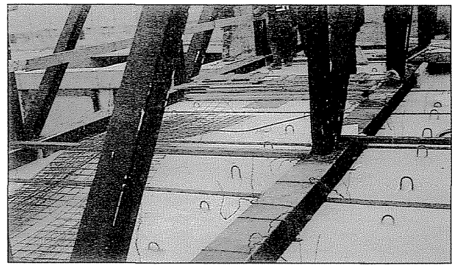
Fig. 8: Floor of the attic (precast)
