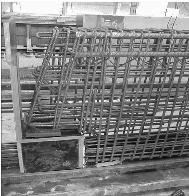
Fig. 6: Reinforcement of the beam type "4000"
