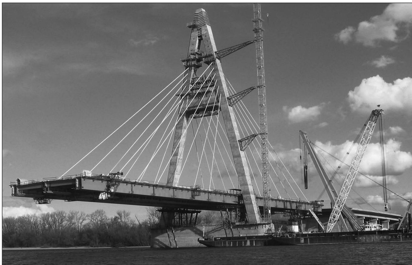
Fig. 4: Parallel construction of the pylons and the deck
