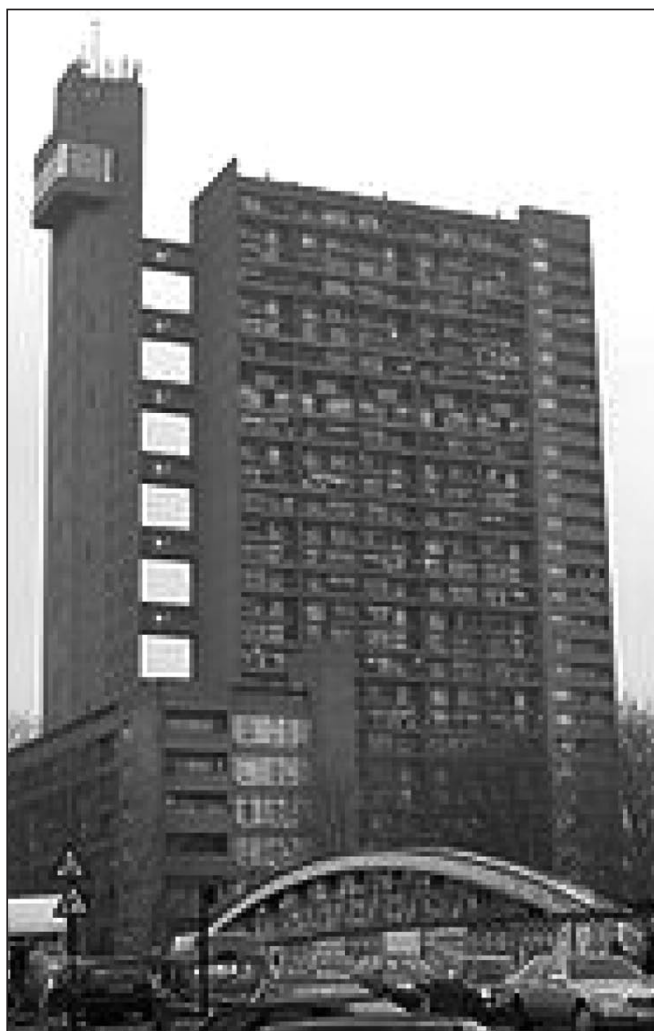
Fig. 16: The Trellick Tower
