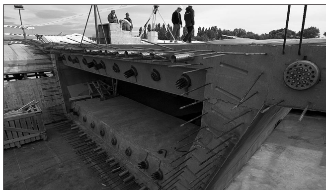
Fig. 3: Cross-section of the construction unit (photo by: György Nyíró)
