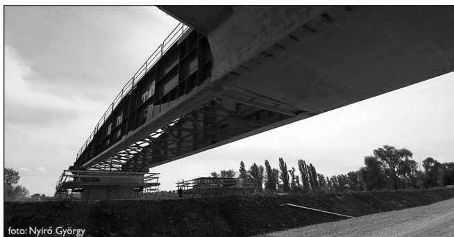
Fig. 4: Steel launching nose (photo by: György Nyíró)
