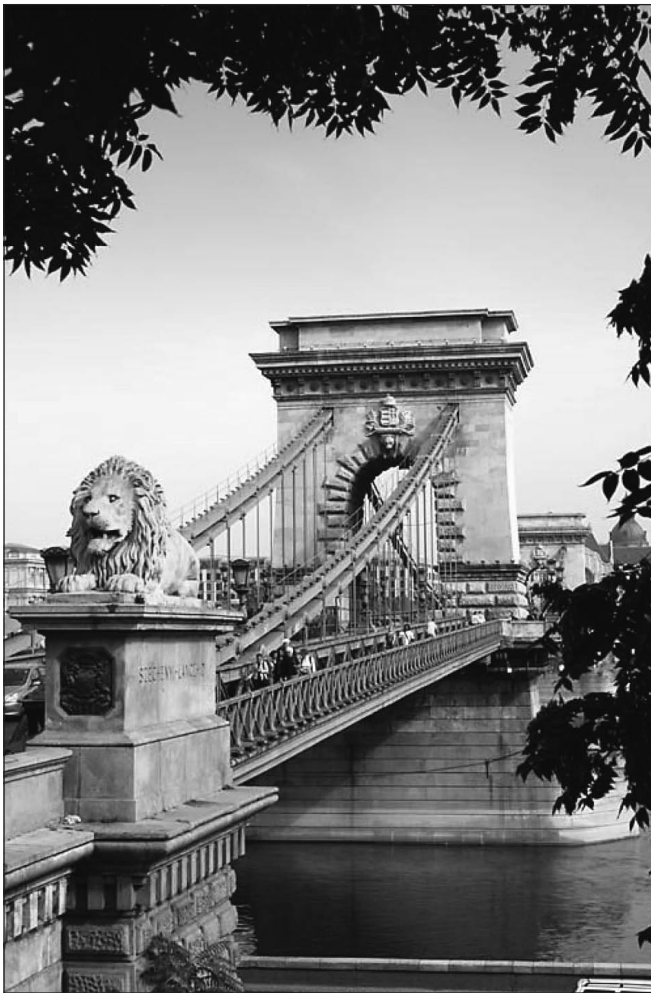
Fig. 10: Széchenyi Chain Bridge
