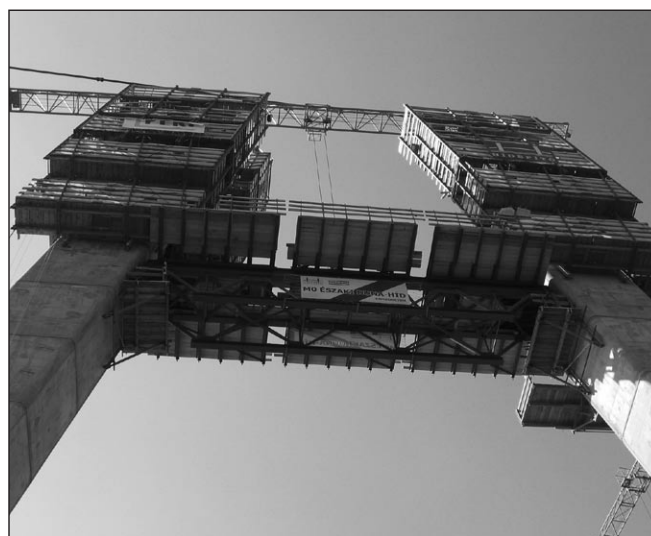
Fig. 3: Pylon construction using the climbing formwork technique
