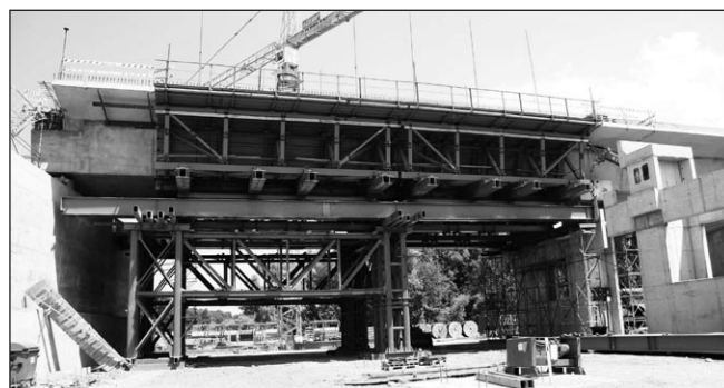
Fig. 5: Casting yard between the piers No. 19 and 20
