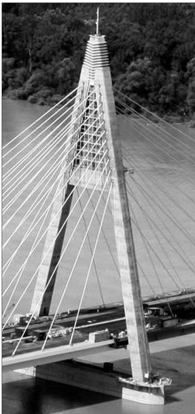
Fig. 2: The "A"-shaped pylon
