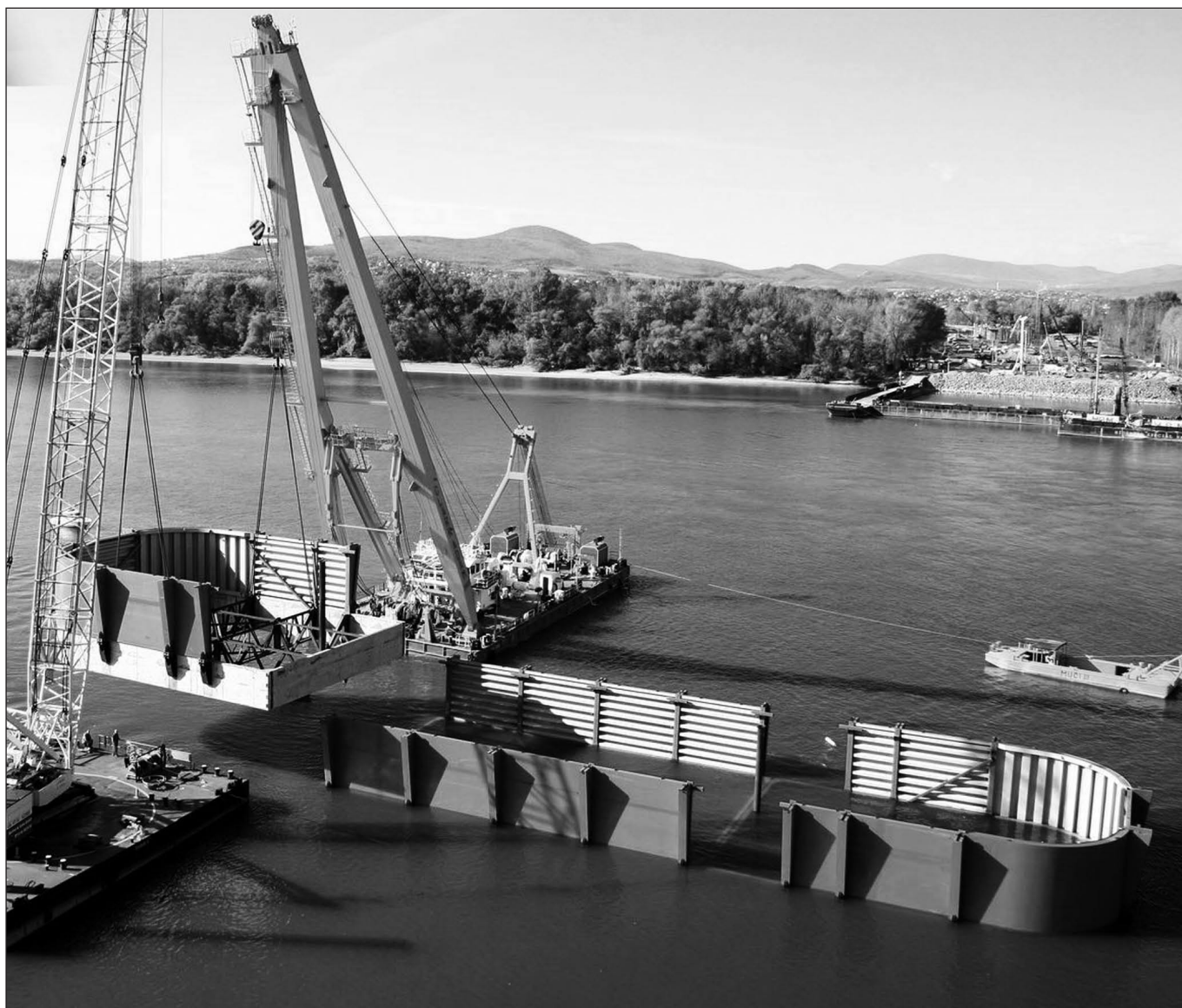
Fig. 1: Positioning of the crib-wall element for the bed pier
