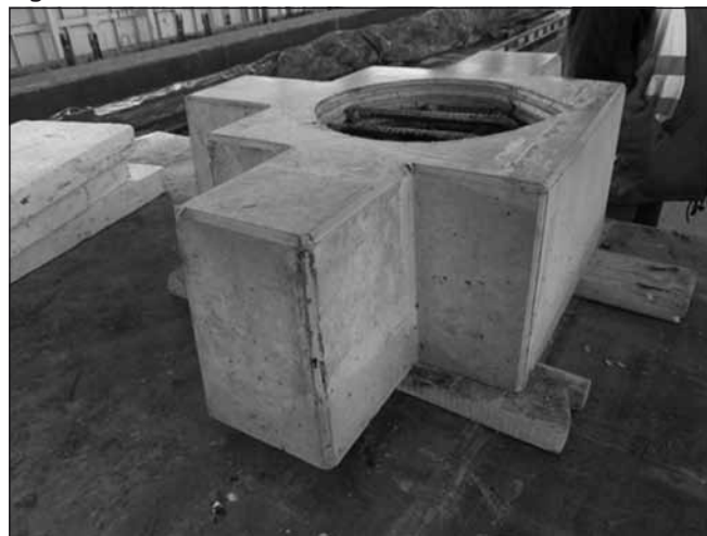
Fig. 11: Precast cantilever bodies
