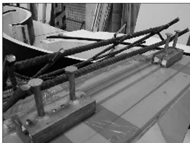
Fig. 4: Steel parts and reinforcement
