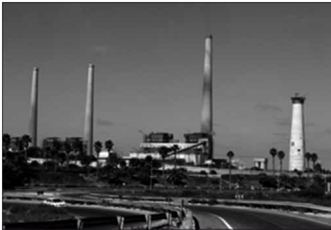
Fig. 10: Orot Rabin site at the Hadera Power Station
