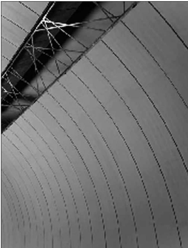
Fig. 7: Mounting of the curved panels
