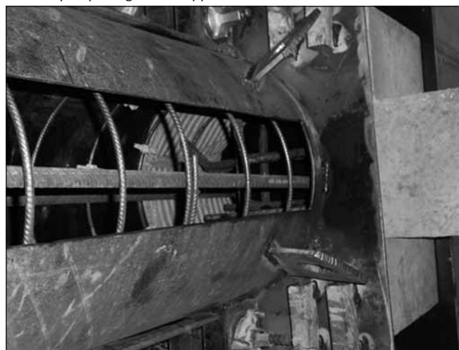
Fig. 12: Horizontal production, the circular formwork has a 12 cm wide stripe opening on the upper side
