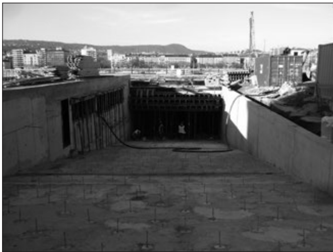
Fig. 12: Built-in, composite action pins with clamping edge in the main entrance ramp on 2nd December 2013
