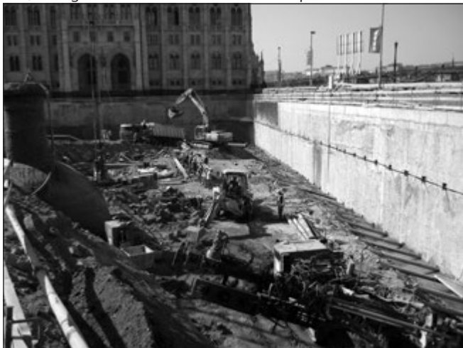
Fig. 5: Earth excavation up to the 2nd anchor level on the Danube side, boring of underwater anchors on 18th April 2013
