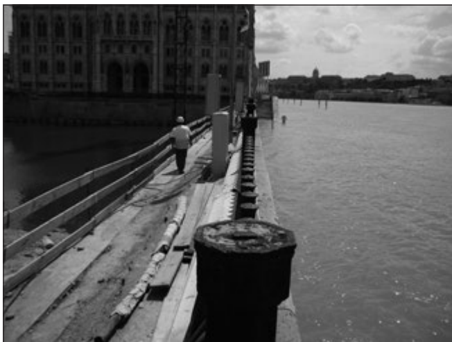
Fig. 7: Artificial flooding measures taken in the construction pit, with a record outside flood on 10th June 2013
