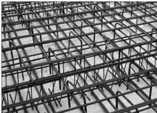
Fig. 15: Crustal concrete poured with white cement decorative concrete and a more dense distance piece steel reinforcement applied at general section to realize composite action of cross section on 5th November 2013
