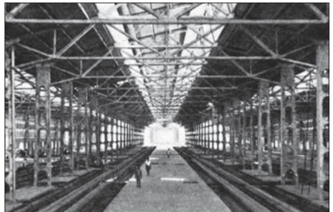
Fig. 31: The erected reinforced concrete structure of a hall
