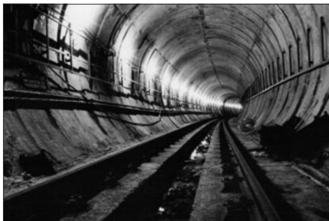
Fig. 24: Interior of the Calcutta metro line under construction
