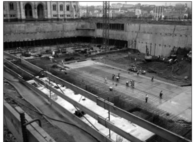
Fig. 6: Base slab completion level before flooding, from Balassi Bálint Street on 30th May 2013
