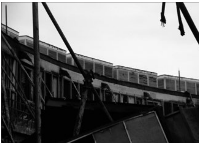
Fig. 2: Destroyed cable heads (ÉMI, 2000)
