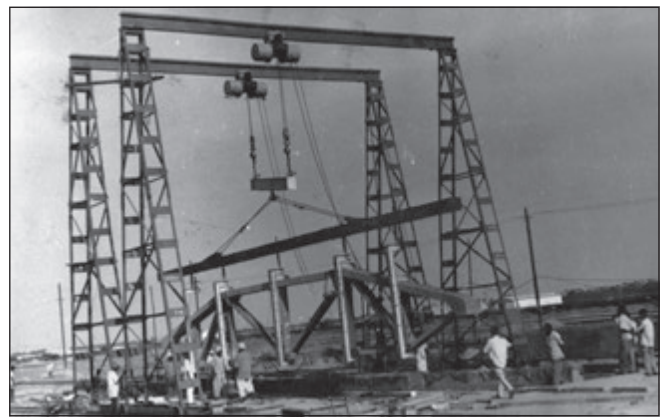
Fig. 30: The site prefabrication
