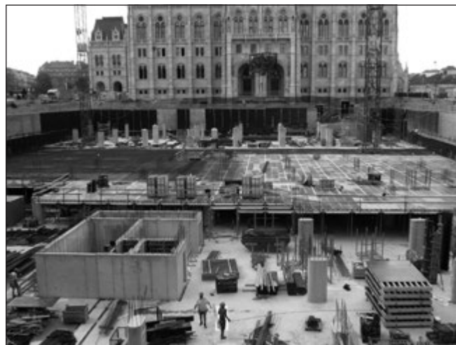
Fig. 8: An intermediate state of construction on 13th August 2013
