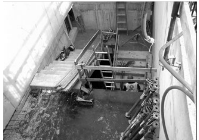
Fig. 13: Built-in and positioned precast flights of stairs on 19th September 2013
