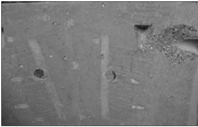
Fig. 8: Tunnel lining after 2 hours hydrocarbon fire
