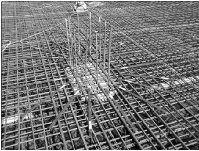
Fig. 11: Puncture type steel reinforcement with radial arrangement in an intermediate slab on 11th July 2013
