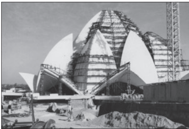
Fig. 13: The Baha'i Temple in New Delhi during construction (1986)
