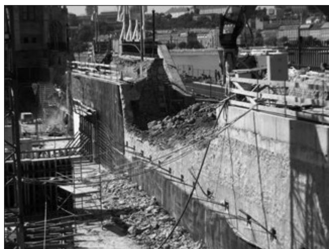
Fig. 9: Demolishing diaphragm wall and upper retaining wall at the entrance to Visitor Centre and deep-level garage on 5th September 2013
