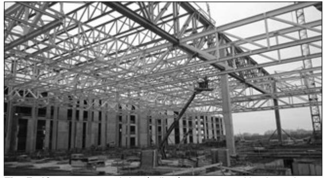
**Fig. 7:** 40 m span truss girders (yellow) are supported by the main truss girders (grey). (ELI 2015)
