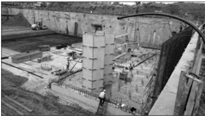
**Fig. 8:** Construction of the basement with varying height. The top and bottom slabs of the basement are connected with groups of honeycomb walls. The height of the basement depends on the weight of the zone above. The weight of the removed soil is close the weight of the superstructure. This method avoids significant settlement and tilt of the building. (ELI 2015)
