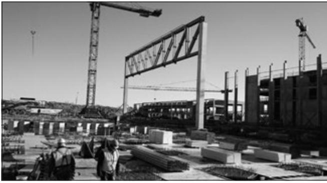
**Fig. 6:** The first pair of main truss girder with a length of 40 m (grey painting) is placed onto the columns of the external structure. (ELI 2015)
