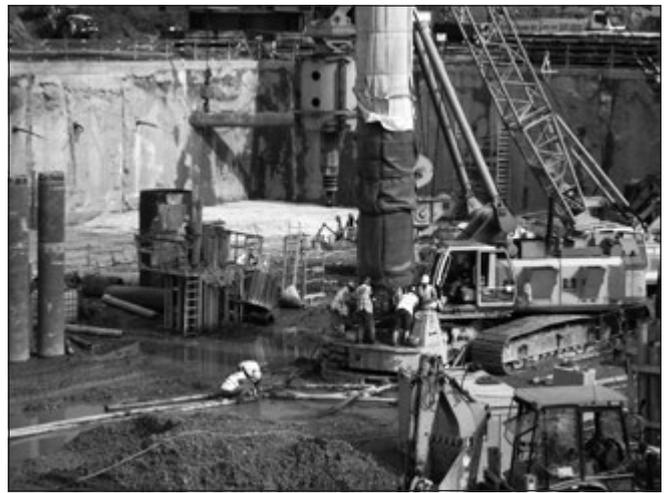
**Fig. 5:** Excavation pit of Building “A” with diaphragm walls and piling under the basement. Erection of a 45 m long central pile using the bentonite-coating technology. The coating avoids the friction along the surface of the pile. The large reaction of the central pile is moved from the reaction zone of the stabilization piles of the basement. (ELI 2015)
