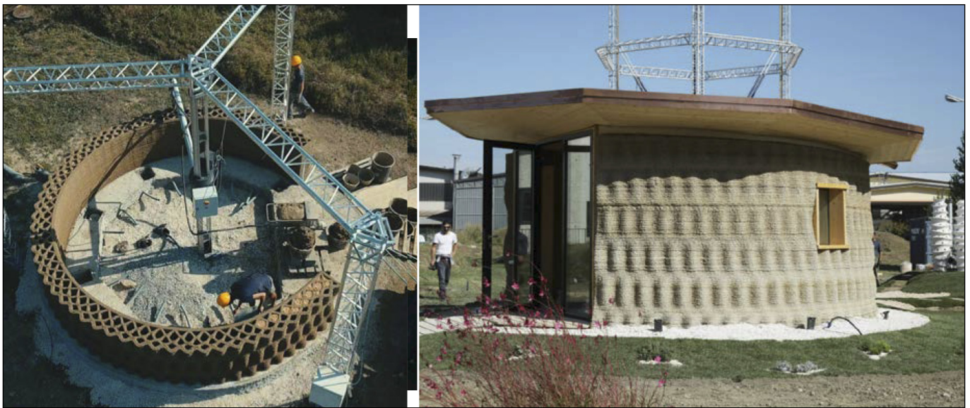
Fig. 3: Gaia house (Gaia, 2018)
