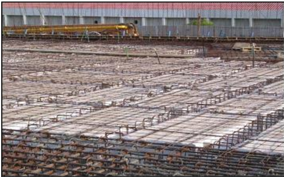
Fig. 4 Polystyrene Blocks with Top Mats in place
