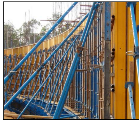
Fig. 3 Formwork for Curvilinear Wall
