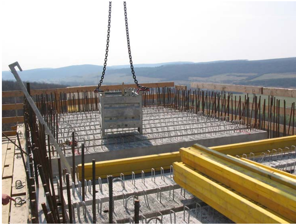
Fig. 9 Prefabricated bridge beams as a formwork for the pier cap beam
