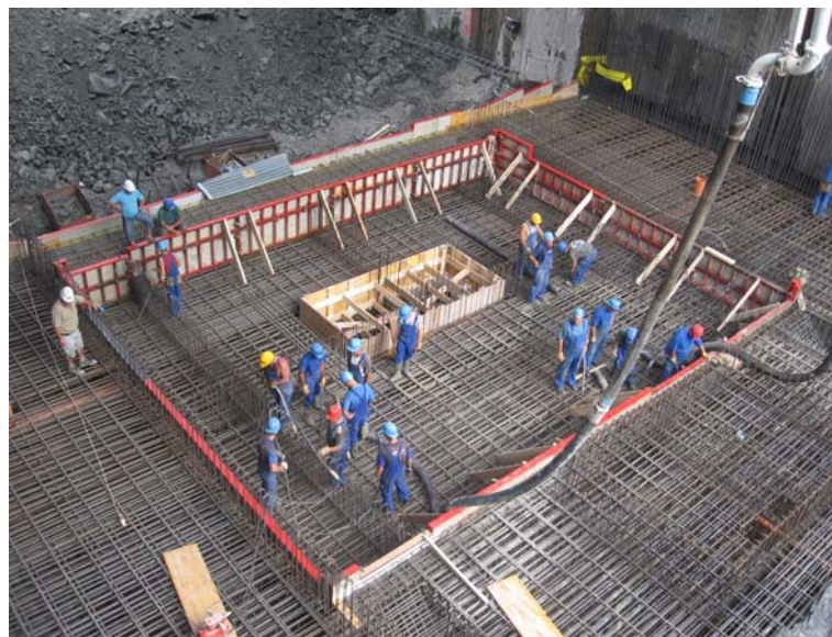
Fig. 7 Construction of bottom slab – concreting blinding concrete, reinforcement
