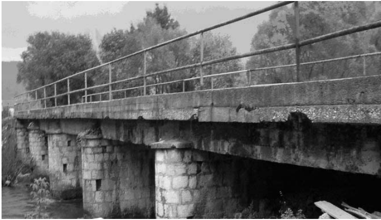
Fig. 4 After the World War II the arch stone structure was replaced by continuous plate
