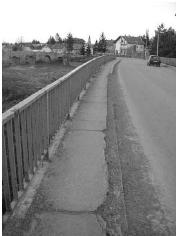
Fig. 6 Deteriorated curbs
