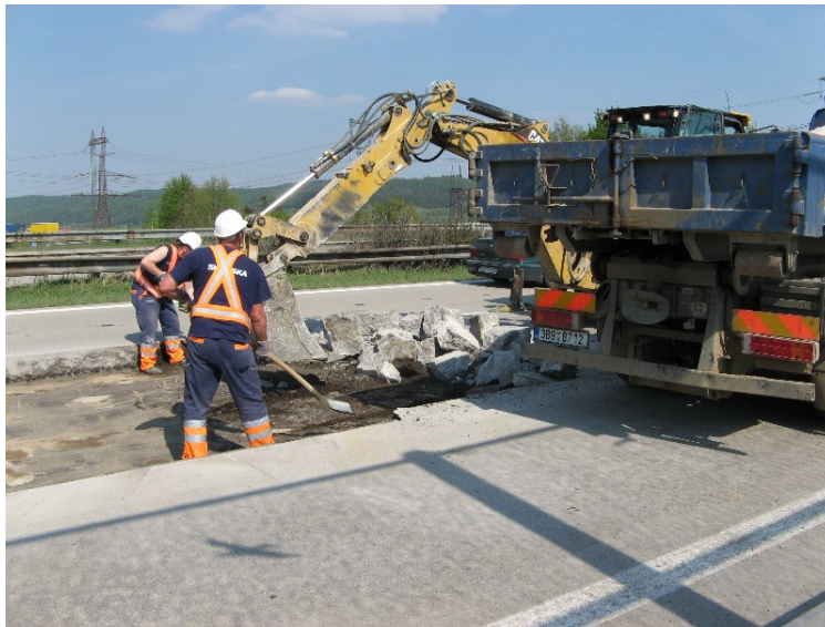
Fig. 1 Removal of damaged slabs or their parts
