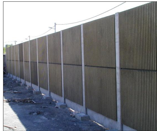
Fig. 4 Constructed noise protection wall
