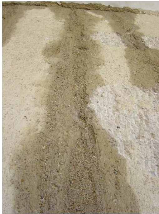
Fig. 1 Rock pockets in a diaphragm wall
