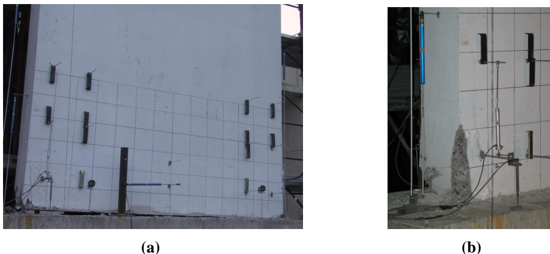
Fig. 4 Details of the single large crack opening at the base of the wall (a) and of the minor spalling of concrete cover in the compressed region (b) at maximum displacement
