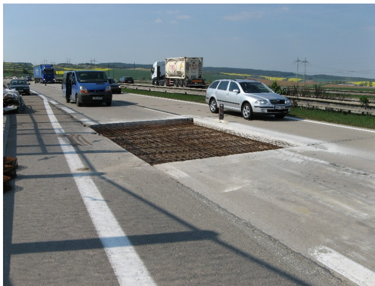
Fig. 2 Reinforcement of new slabs
