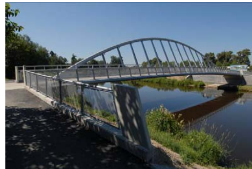
Fig. 14 Composite deck suspended pedestrian bridge across Vltava river in Ceske Budejovice
