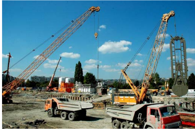
Fig. 4 construction of diaphragm wall
