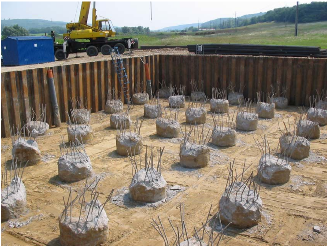
Fig. 3 Bored piles and the sheeting for the pile cap
