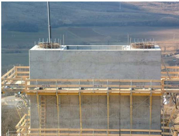
Fig. 10 Completed pier cap beam
