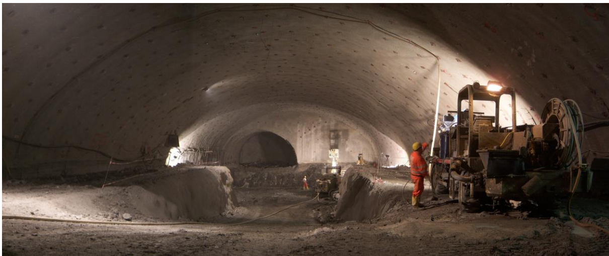
Fig. 8 Section „East”, Widenig before twin tunnel
