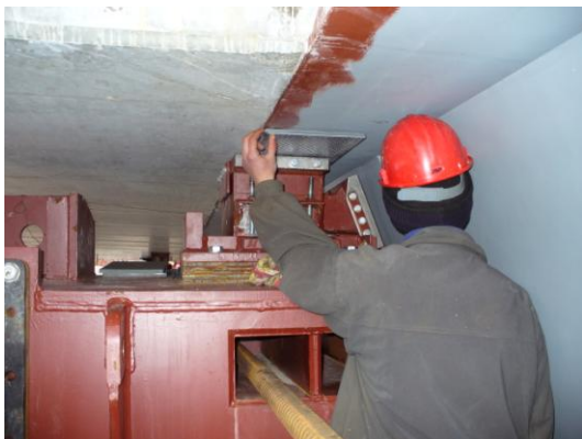
Fig. 6 Sliding bearing
