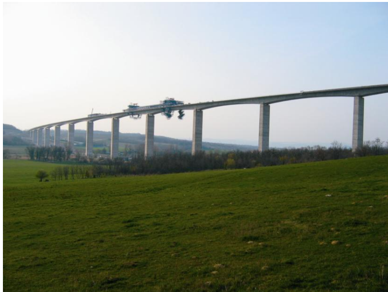
Fig. 13 Viaduct on the M7 motorway at Kőröshegy (Wellner, Mihalek, Barta, 2005)
