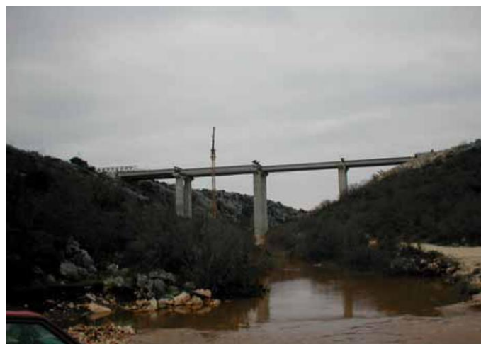
Fig. 4 Appearance of the Kličevica Bridge in construction
