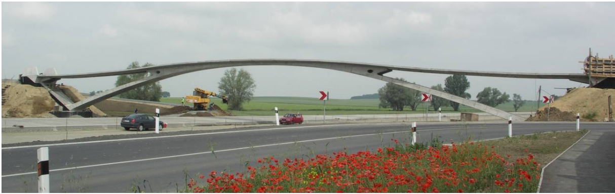
Fig. 9 After placing the segments
