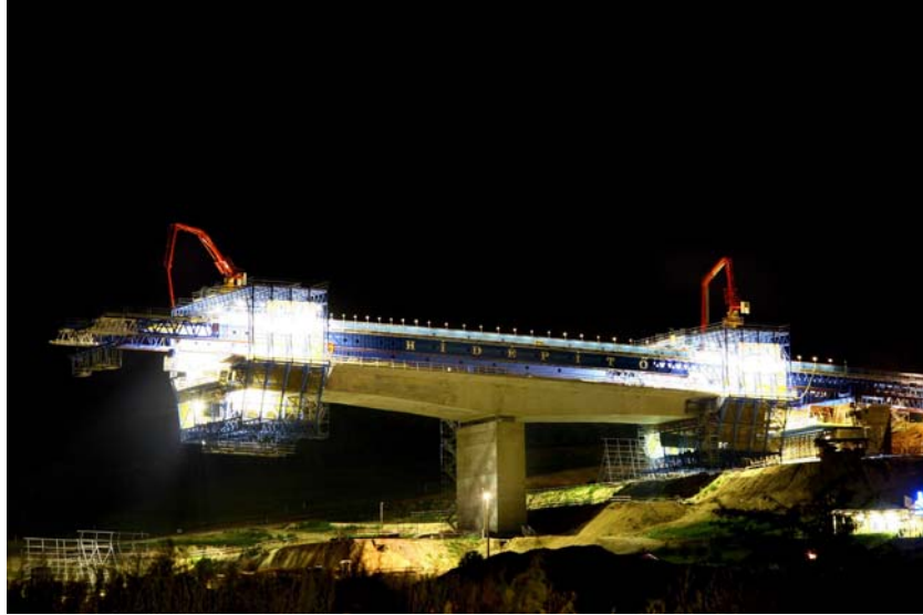
Fig. 2 Construction of the superstructure
