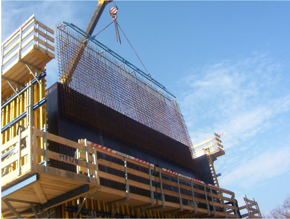
Fig. 6 Lifting of the prefabricated reinforcement into the formwork
