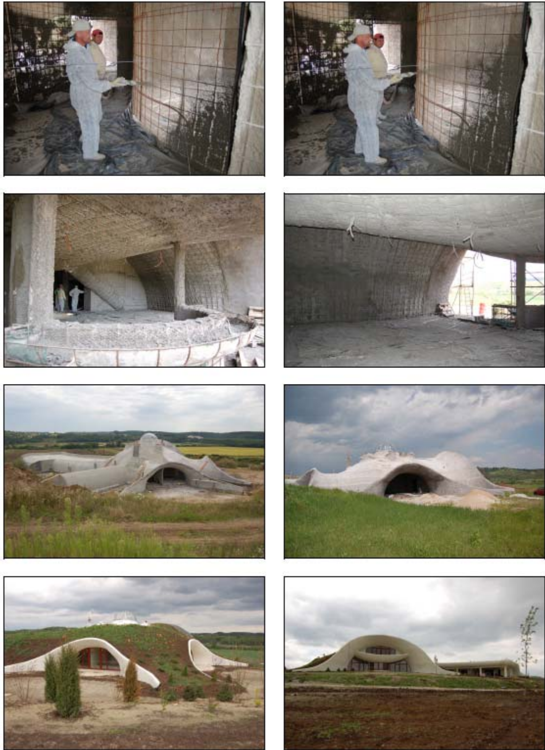
Photo 7 Inside and outside surfaces of the structure under and after construction together with the views of the building
