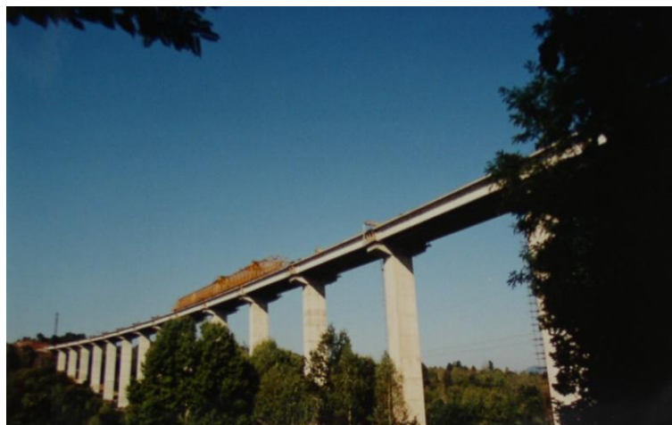
Fig. 2 Appearance of the Severinske Drage Viaduct in construction
