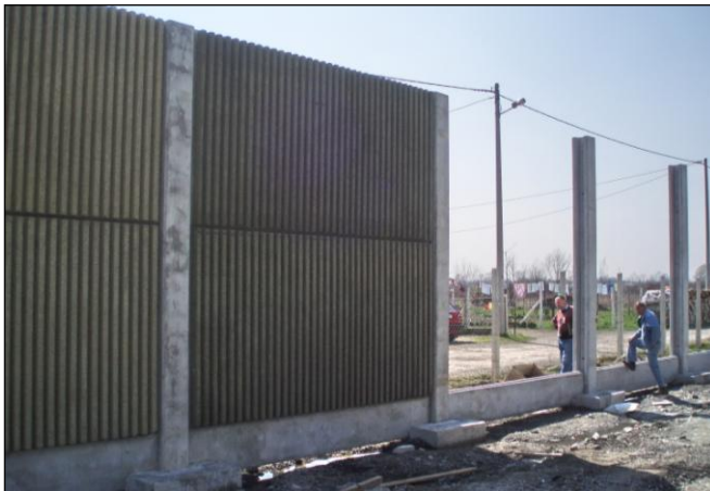
Fig. 3 Building of the noise protection wall
