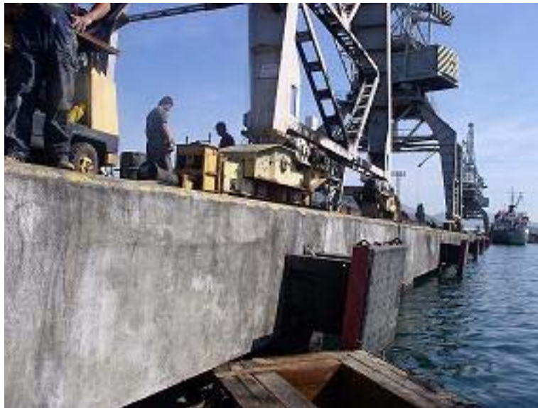
Fig. 1 The module No. 3 in port Ploče
