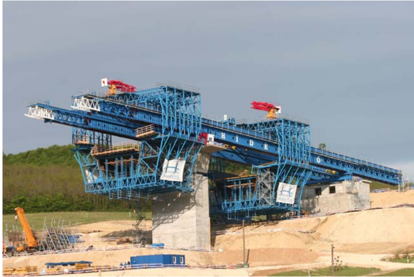
Fig. 1 The auxiliary structure
