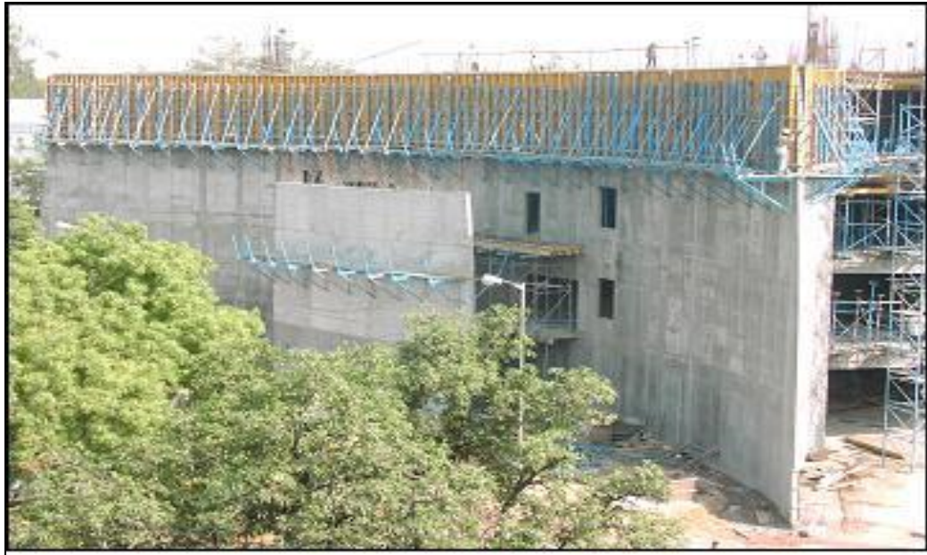
Fig. 5 View of Curvilinear Wall
