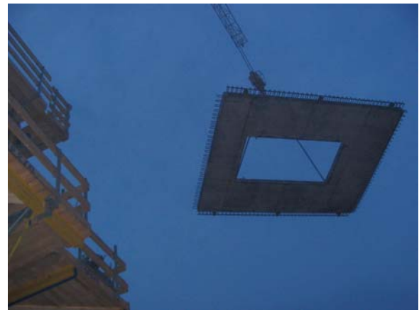
Fig. 8 Lifting of the diaphragm
