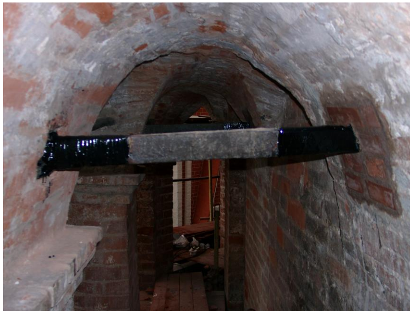
Fig.1 Strengthening of metal tension bars in brickwork vaults with carbon fibre anchors, St. Basil's Cathedral, Moscow
