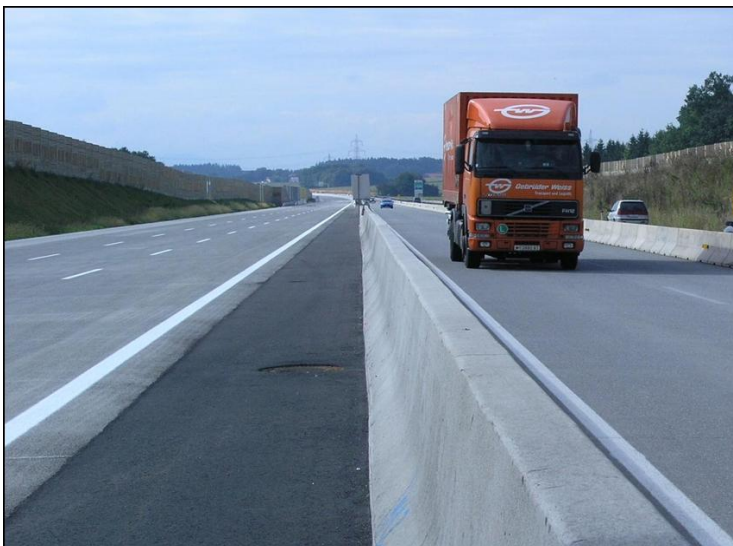
Fig. 1 Difference between bright concrete pavement respectively bright guide wall and dark bituminous surface
