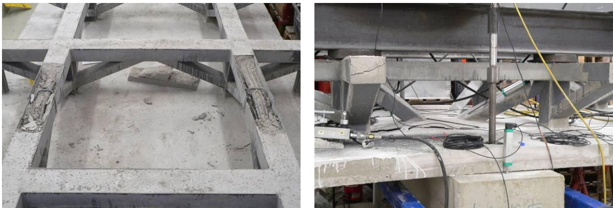
Fig. 8 The failure of specimen 2 after ultimate load
