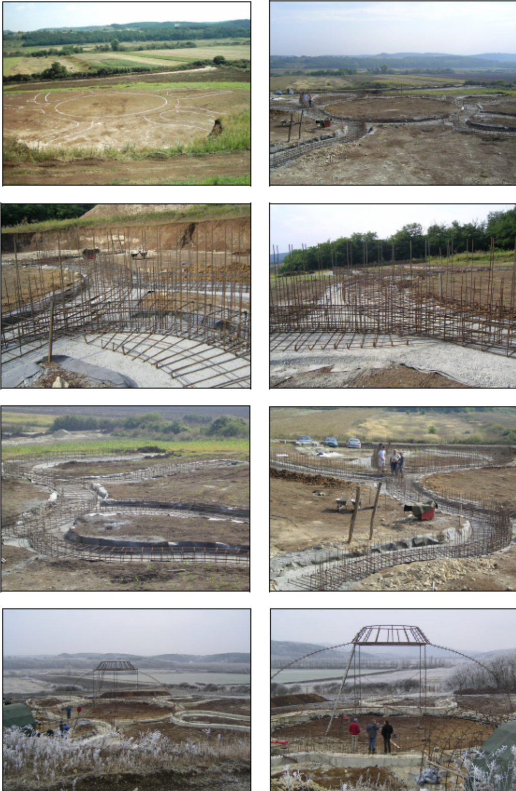
Photo 5 Construction of foundation and the steel tube "skeleton"
