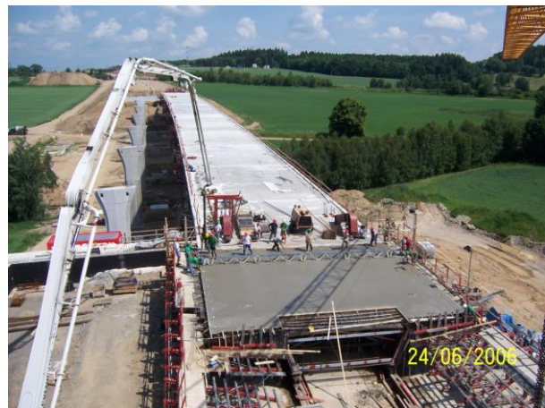
Fig. 9 Casting of the 18 m long segment
