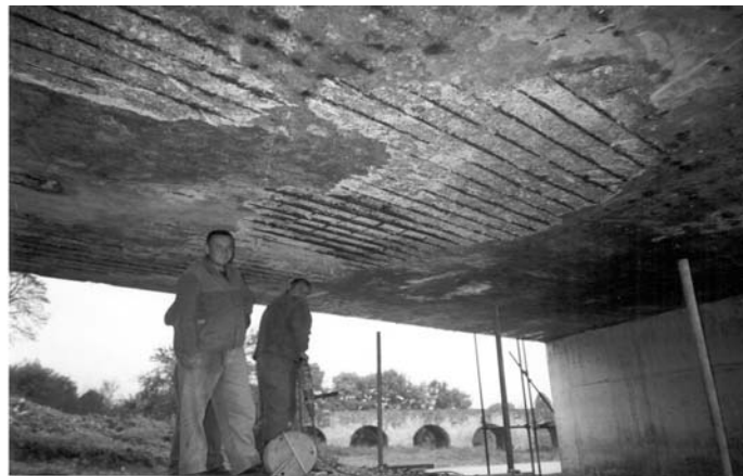
Fig. 7 Deteriorated lower side, bridge Oštarije
