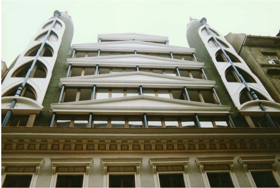
Fig. 5 Glass metal FRC folded plate elements with 20 mm thickness
