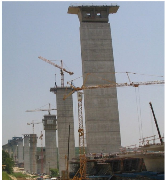
Fig. 5 Piers under construction
