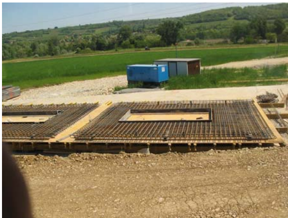
Fig. 7 Reinforcement of the diaphragm
