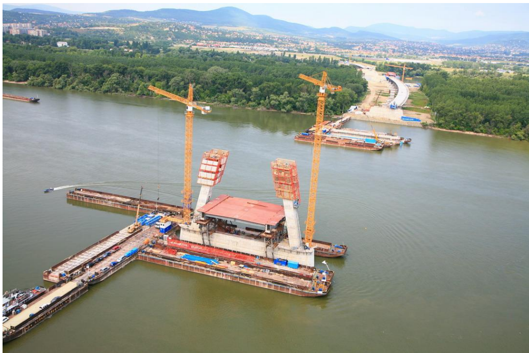
Photo 2 Construction of pylons with using climbing shuttering technology
