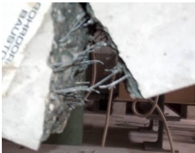
Fig. 2 Failure with fibre pull-out
