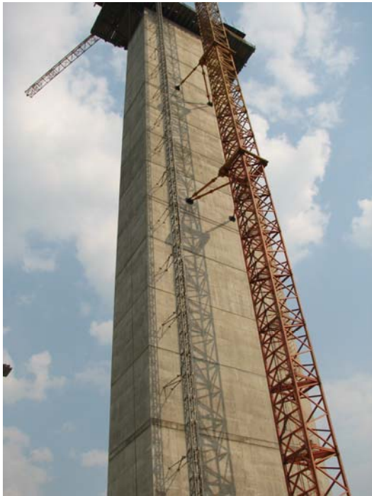
Fig. 12 Pier 7. with 100 m tall crane
