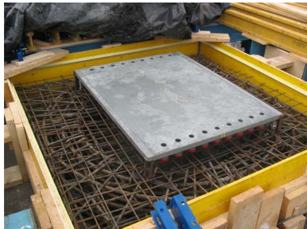
Fig. 11 Bearing bottom plate in the formwork
