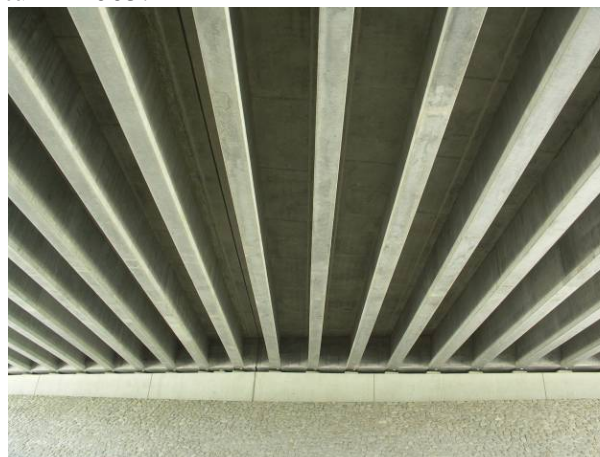
Fig. 2 Precast girders and composite slab
