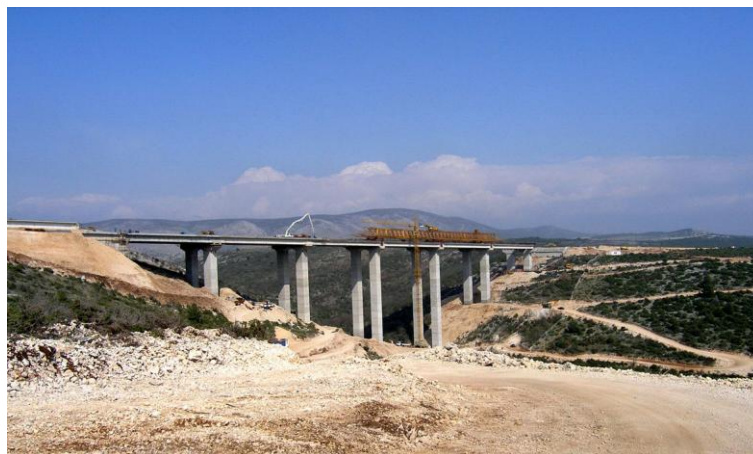
Fig. 6 Appearance of the Dabar Bridge in construction
