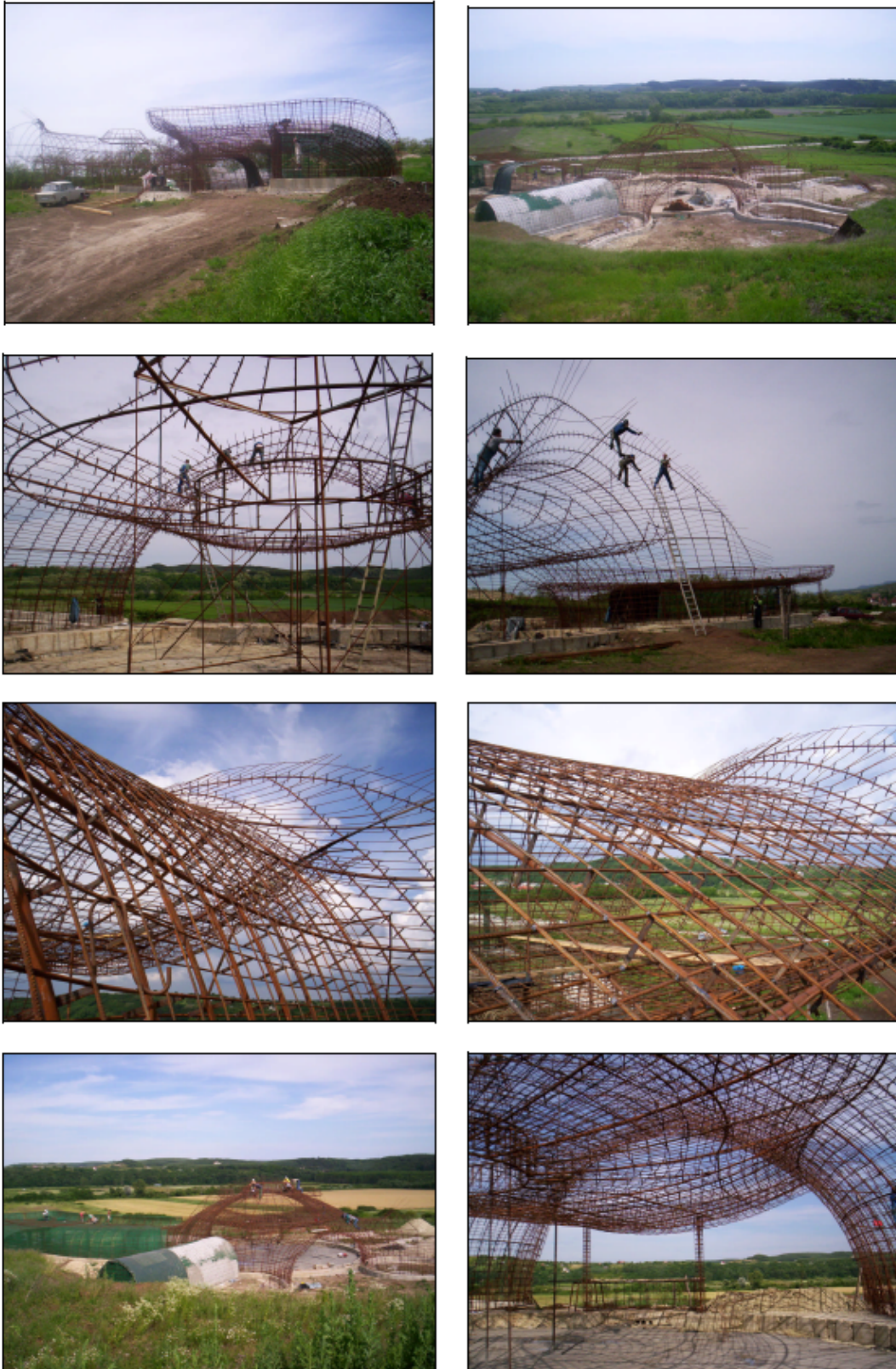
Photo 6 Release of the double reinforcement meshes on the prefabricated steel tube "skeleton"
