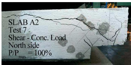
Fig. 9 Slab A2 with hooks and bent-up bars: Test No.7, concentrated load, P_u = 383 kN
