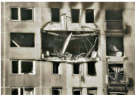
Fig. 2: Explosion damage in Budapest
