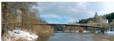
Fig. 3 Chain bridge (CZ)
