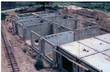
Fig. 3 Mounting of Panel Elements with the Aid of Sleeve Splices
