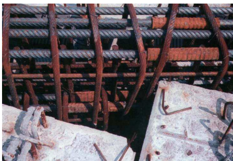
Fig 4 Splicing of the reinforcement in a concrete bridge
