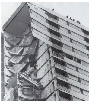
Fig. 1: Ronan Point collapse
