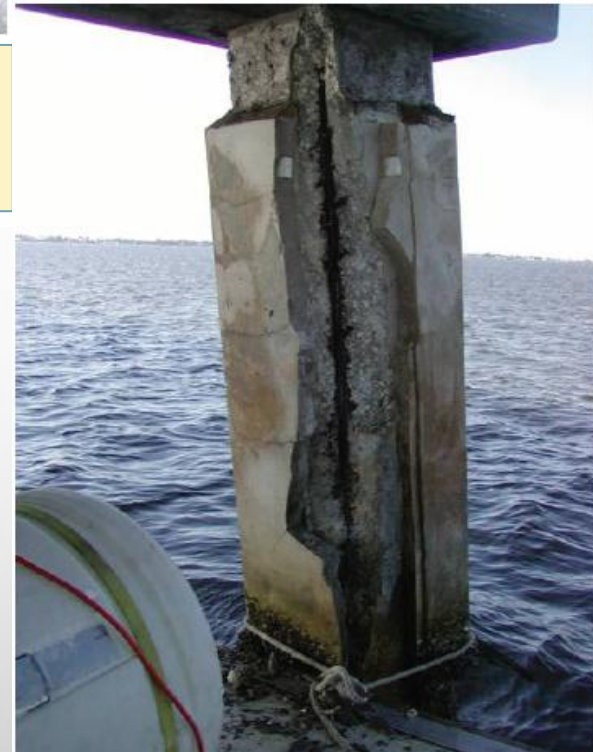
Figure 2.40. Marine pile degradation: (a) jacket failure Source: Courtesy Atkins North America, Inc.
